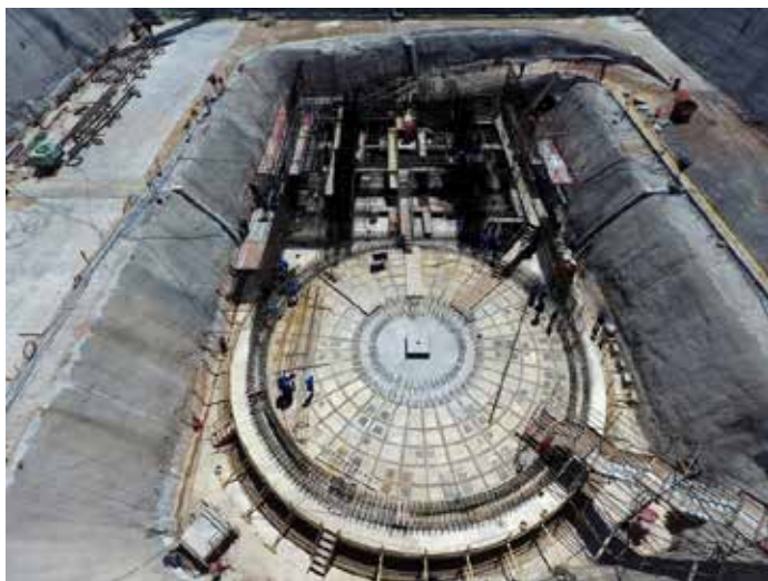
The CAREM SMR under construction in Argentina.
